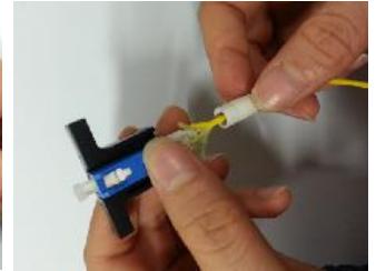
4/ Divide Kevlar into 2 equal portions and screw the lock nut onto back of connector to secure Kevlar tightly. Then, slide the boot up. (If for 250 or 900µm cable, jump to point 5)
