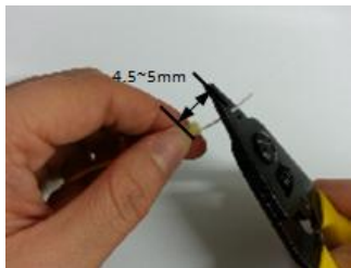
4/ Strip 900µm primary coating off and leave 4.5~5mm of 900µm buffered fiber.
